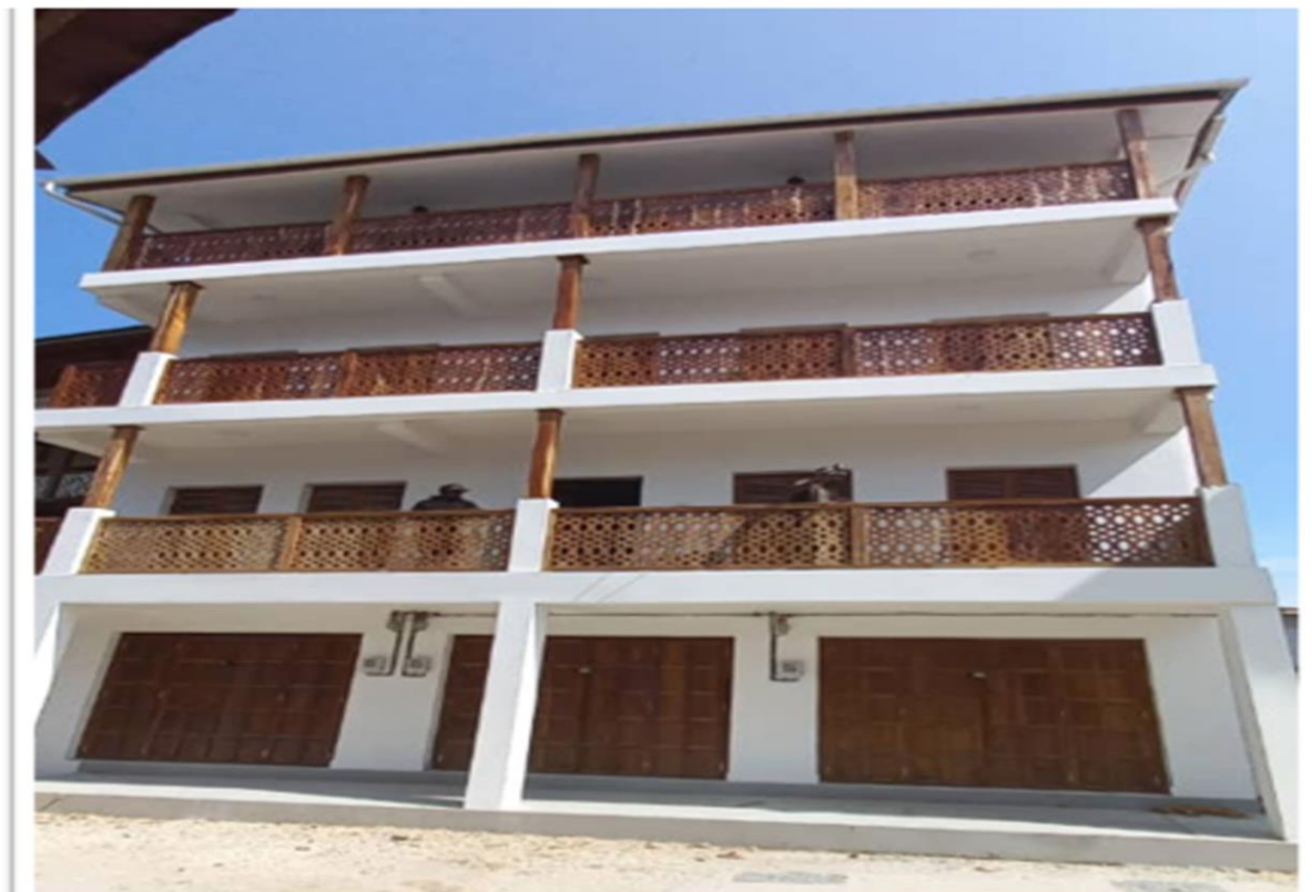
The completed building features fully installed balustrade panels, providing both aesthetics and safety
