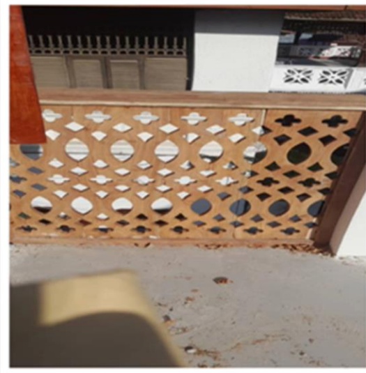
The building is in the early stages of balustrade installation
